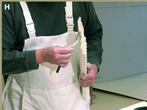
H Apply adhesive to the cornice mitre
