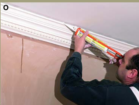
O If required the ceiling and wall lines can be filled with decorators caulk
