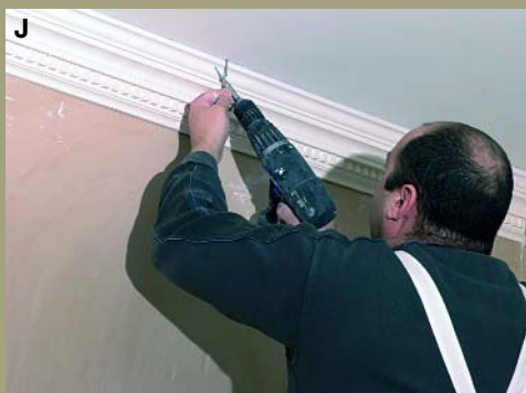
Fixing the screws
