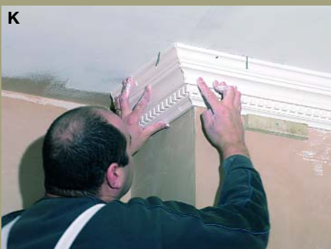
K Position the cornice mitre joint
