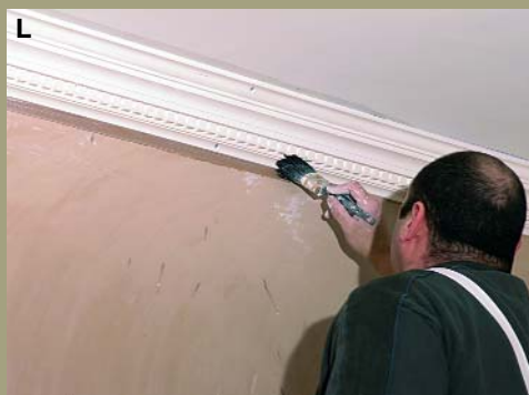
L A small paint brush can be used to wash in the ceiling and wall lines
