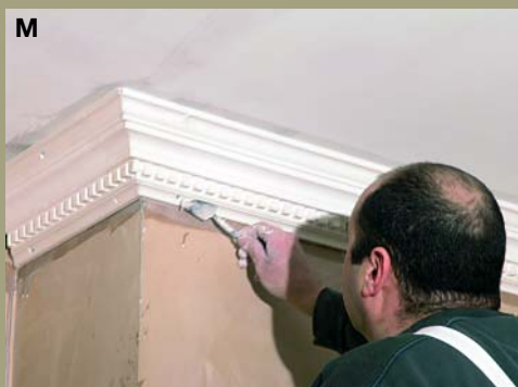
Fill over screw heads
