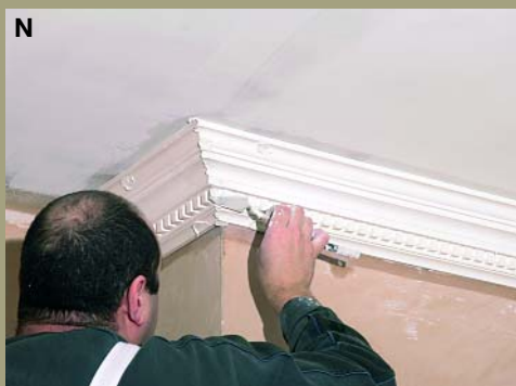
The joint rule and small tool can be used to fill mitres or knife off the excess
